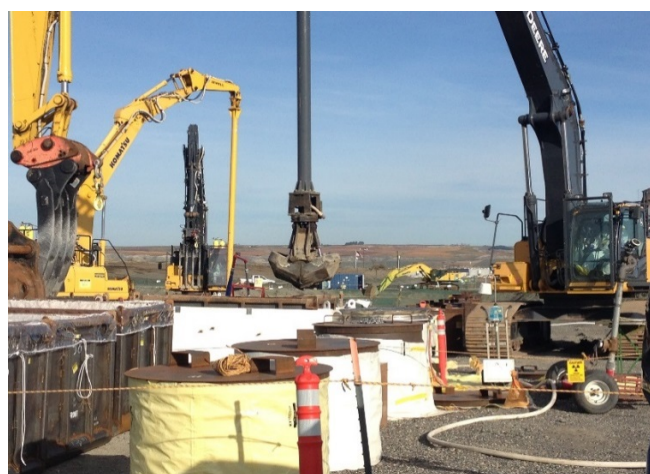
Fig. 10. VPU Waste Retrieval Clamshell.
