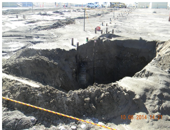
Fig. 3. VPU Potholing.
