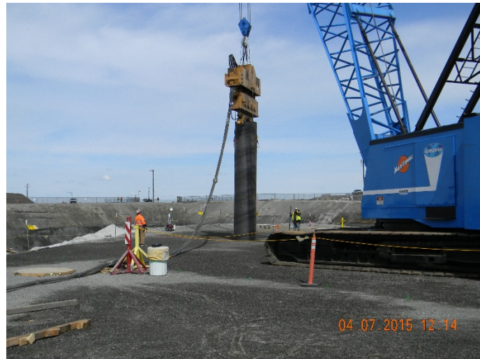
Fig. 6. Installation of Over-Casing.
